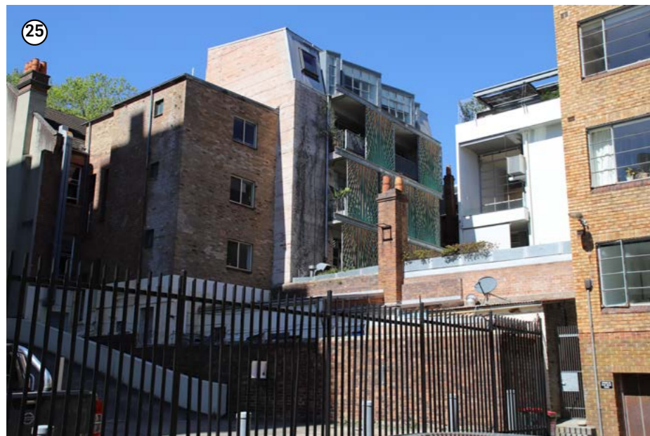
Plate. 26 Detail view of western elevation (rear facade) of 57-59 Macleay Street
