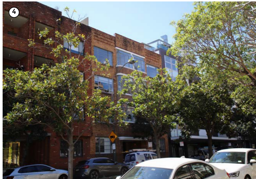
Plate. 4 Detail view of 10B and 10C Challis Street south of the subject site
