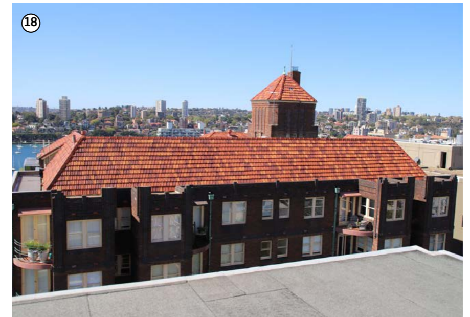
Plate. 18 View east to 10-12 Macleay Street from south-east corner of the subject sites' rooftop
