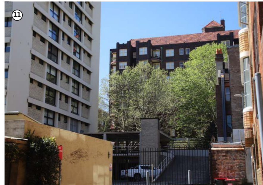
Plate. 11 View towards Macleay Street from McDonald Lane near the south-western corner of the subject site
