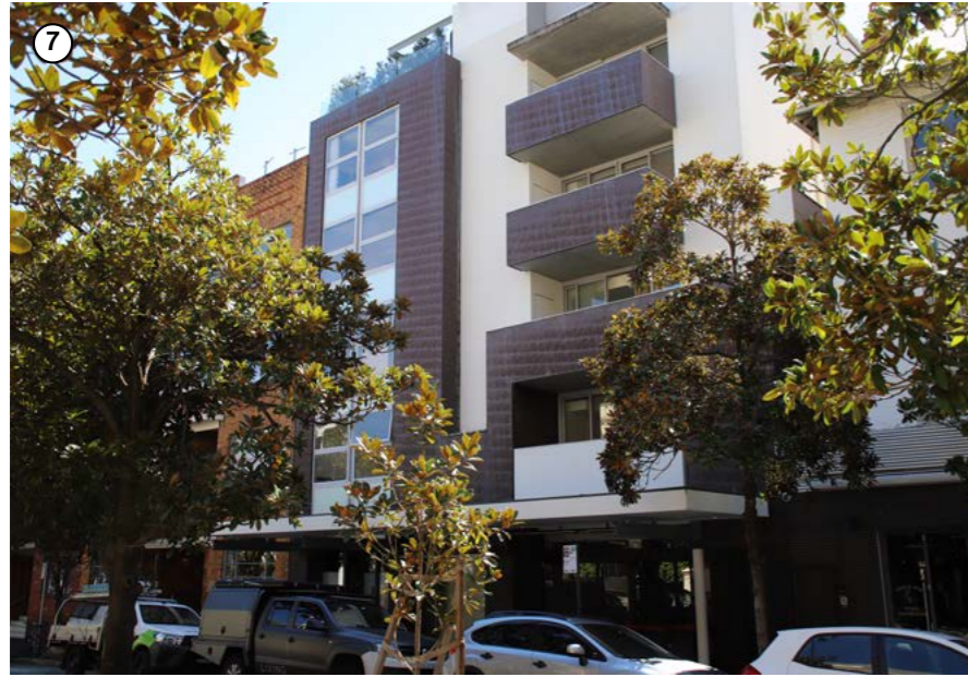
Plate. 7 Detail view of 14 Challis Street south of the subject site
