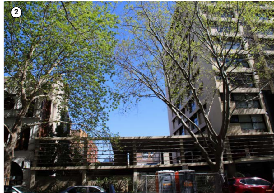
Plate. 2 View west from Macleay Street towards southern setback of the subject site
